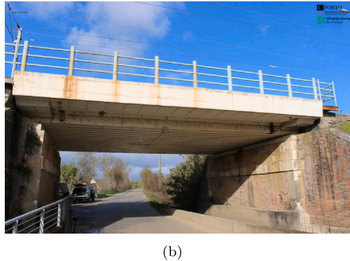
Fig. 10. Cascalheira underpass. (a) cross-section (unit: m); (b) view of the deck.
