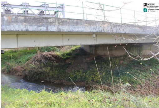
Fig. 9. Melga bridge. (a) cross-section (unit: m); (b) view of the deck.
